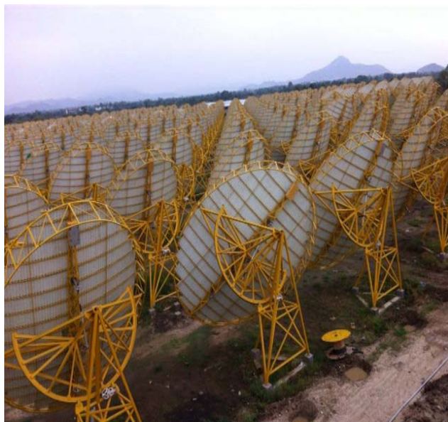
Fig. 5: Electricity generation using scheffler reflector
