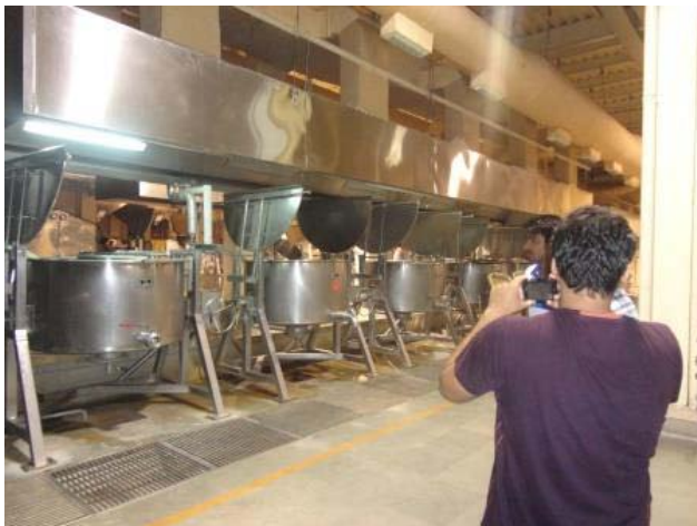
Fig. 3: Steam cooking by scheffler reflector at Shantivan complex (Abu road)
